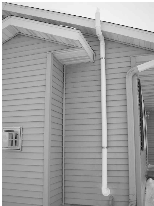
Figure 10 – Vent Line Installation
