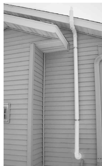
Figure 9 Vent Line Installation (3 inch)
