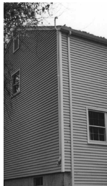
Figure 8 Vent Line Installation (2 inch)
